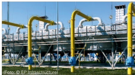
(Foto: © EP Infrastructure)
